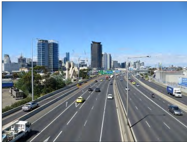
Ingles St Bridge (top) View from Ingles St Bridge (bottom)
